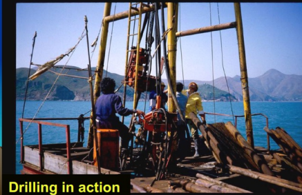
Drilling in action
